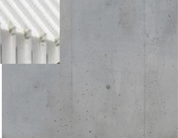
EF03 Off-form concrete
